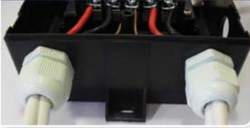
**4** Connect wires to geyser's connector block.
