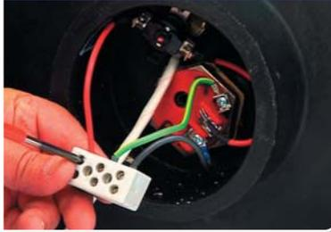
**5** Push the plug connected to the geyser temperature probe through the hole as provided on the geyser.
