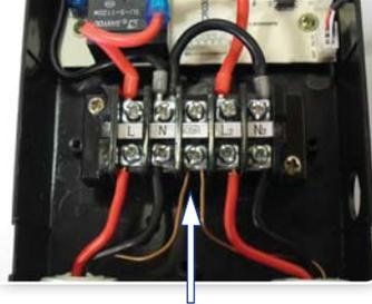
**Connect the wire from isolator to controller**
